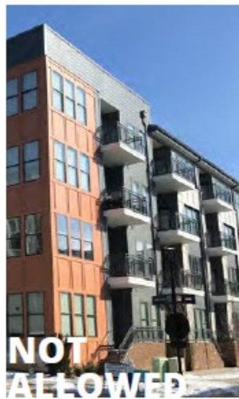
Balconies: Extending Off Façade
