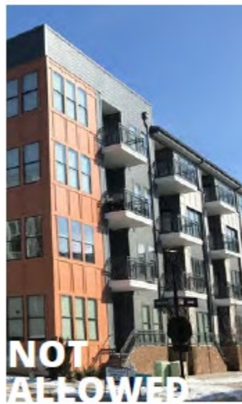
Balconies: Extending Off Façade
