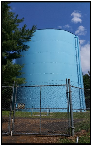
West Ground Storage Tank
