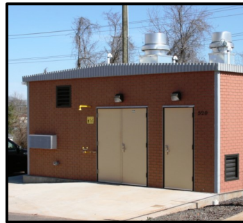
Well System Treatment Building
