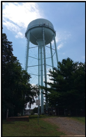
Elevated Storage Tank
