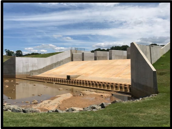
Mountain Run Lake Dam
